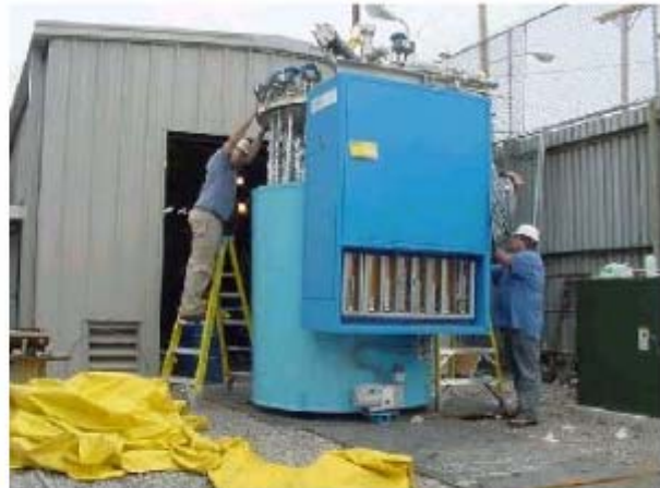
Refrigeration system for superconducting cable.
