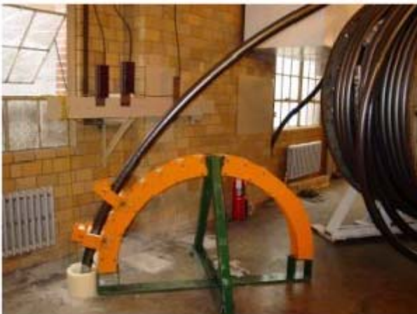
Superconducting cable being pulled in underground circuit.
